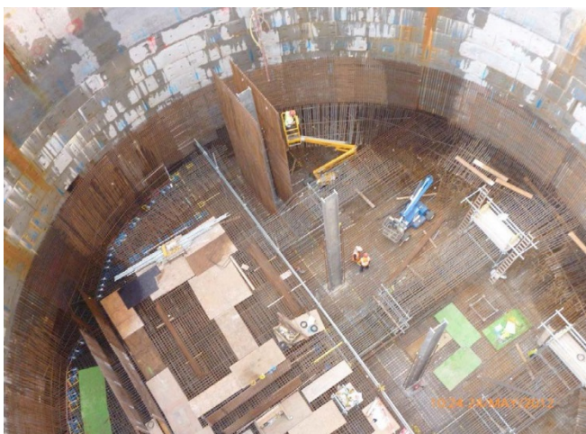
Plate B10 – Wall starter bars installed and fixed to structural steel. Additional structural lacer bars fixed at top of wall to distribute loads back to the post
