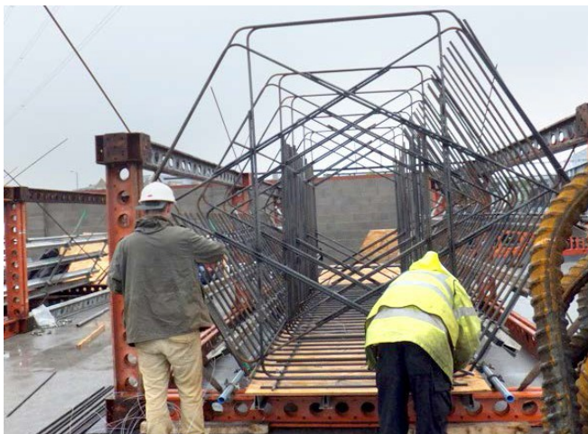
Plate B2 – Opposite end of jig showing alignment rails
