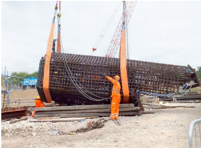
Plate B6 – Cage rotated using appropriate lifting equipment
