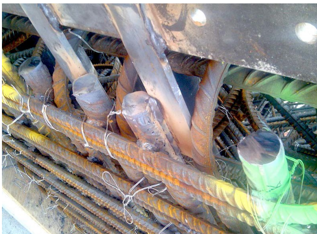
Plate B5 – Detail of welding lugs fixing the template to the front of the cage
