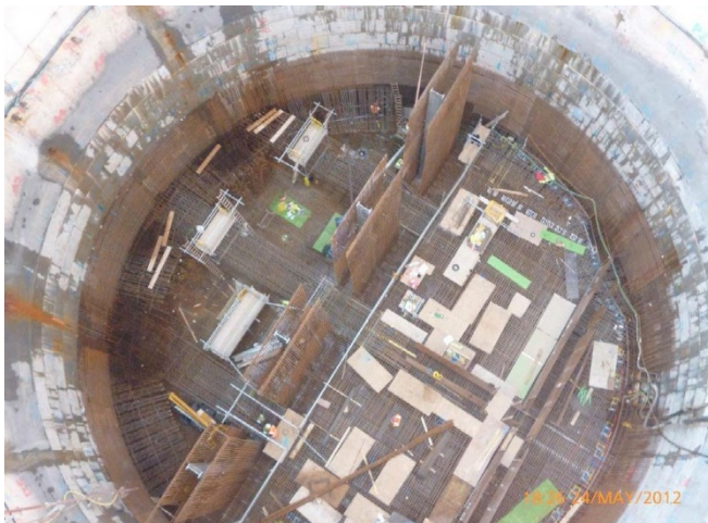
Plate B12 – Wall starter bars installed in preparation for base slab pour
