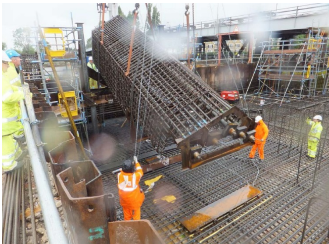
Plate B7 – Cage lifted into position
