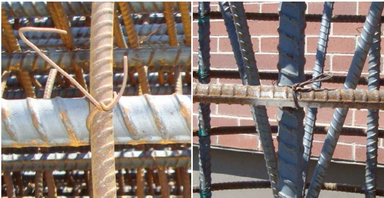
Plate 5.1 – (Left) Single slash tie (Right) Double slash tie
