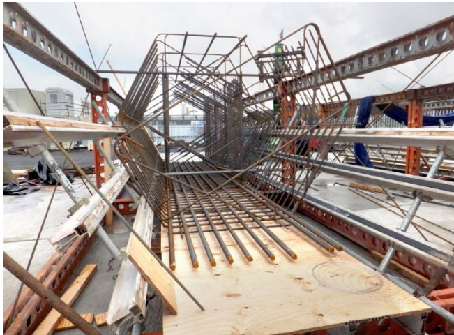
Plate B1 – Initial fixing in an offsite jig
